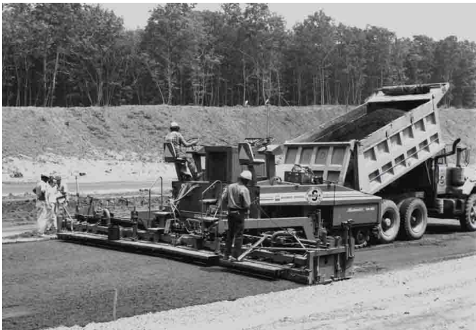
This Matmaker asphalt finisher uses a Screw Conveyor at the back of the tractor unit to move material outward in both directions and spread it uniformly across the entire paving width.
